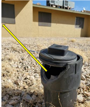
Outdoor Odors from Broken Clean-Out Caps or Missing Clean Out-Caps
