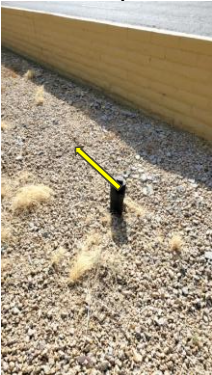
Outdoor Odors from Broken Clean-Out Caps or Missing Clean Out-Caps
